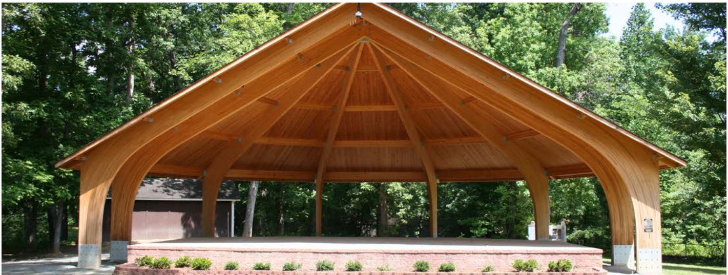
The glulam framework shows an intricate design that would not be possible with regular wood. Photo courtesy of Structural Wood Systems (SWS).
