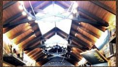
The simple scissor trusses add an understated elegance to the structural design.
