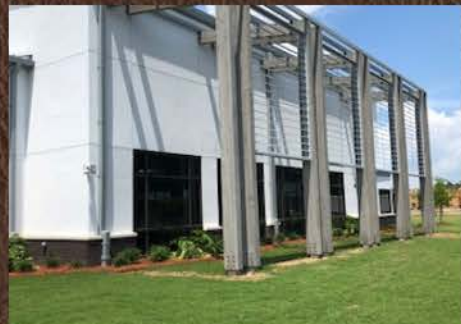
The finish on the exterior glue-laminated members compliments the exterior finish of the new school.
