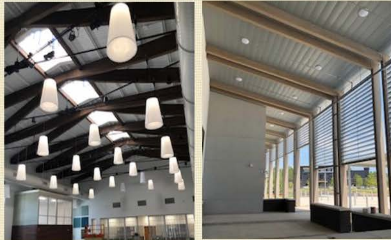
The tie rod assemblies are attached to the glulam frames using SWS custom semi-concealed connections.
