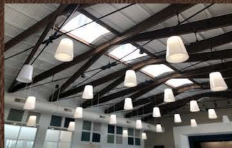
The glulam frames feature a dark stain which provides a rich contrast with the natural light in the cafeteria area.
