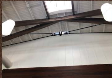
The tie rod assemblies are attached to the glulam frames using SWS custom semi-concealed connections.
