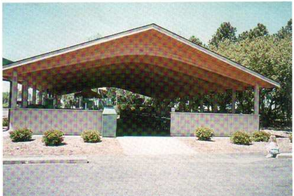
Shelter Building, Michigan State University, East Lansing, MI.
