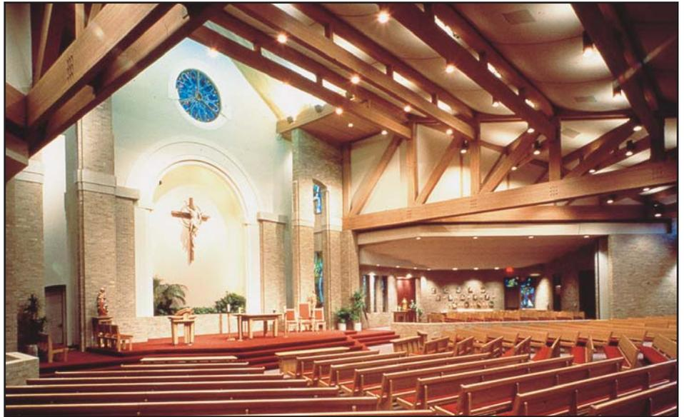
The main glued laminated structural trusses support other laminated beams connecting at various angles with special fabricated connections. Top and bottom chords of the two main trusses have double 6-3/4 in. x 30 in. members to add visual interest.
